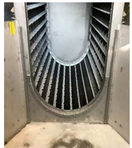
View in the channel during installation
