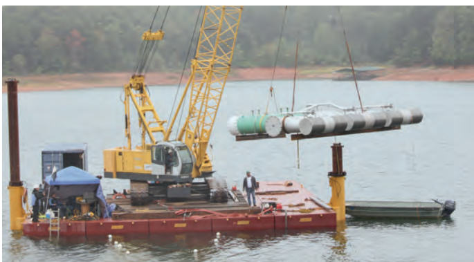
Johnson Offshore Intake Systems™ (JOIS™) Installation
