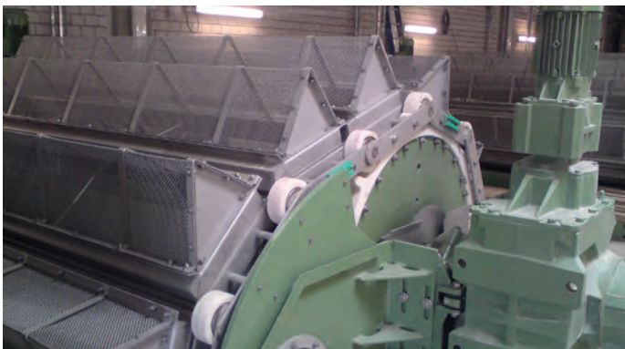
Geiger® Centre-Flow Travelling Band Screen
