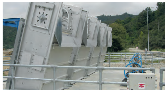
Geiger® High-Capacity Revolving Chain Screen
